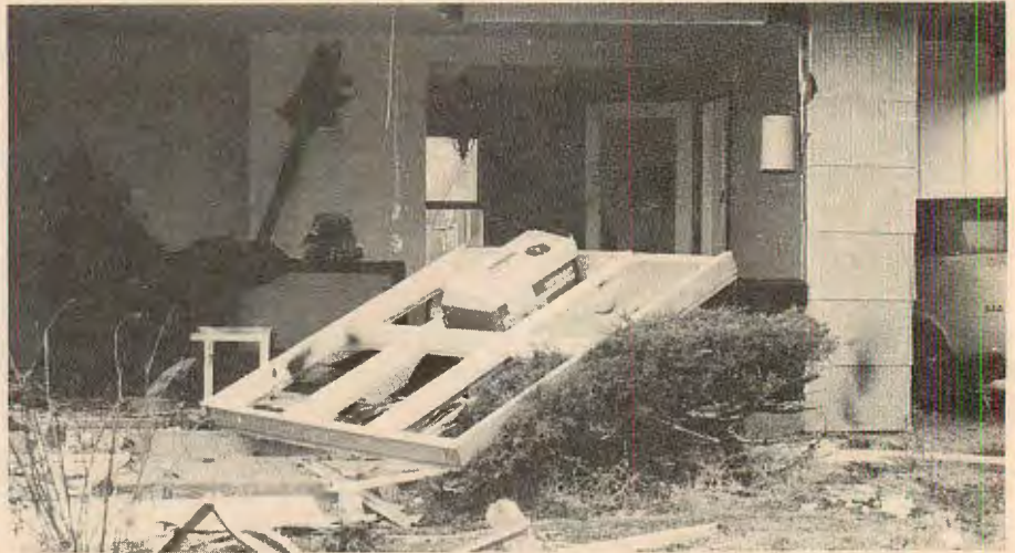
Gunman's house, showing effectiveness of tactical unit's battering ram.
